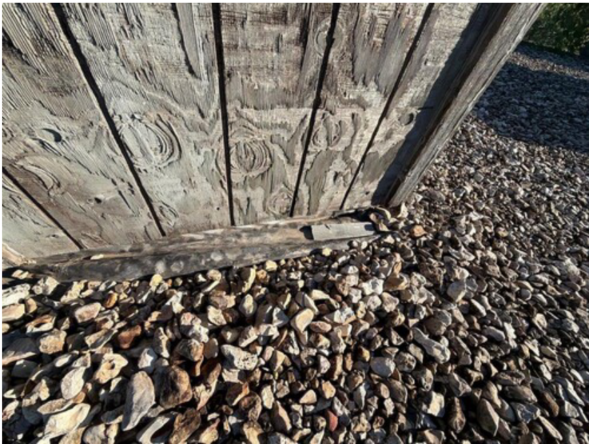
Major chimney deterioration
