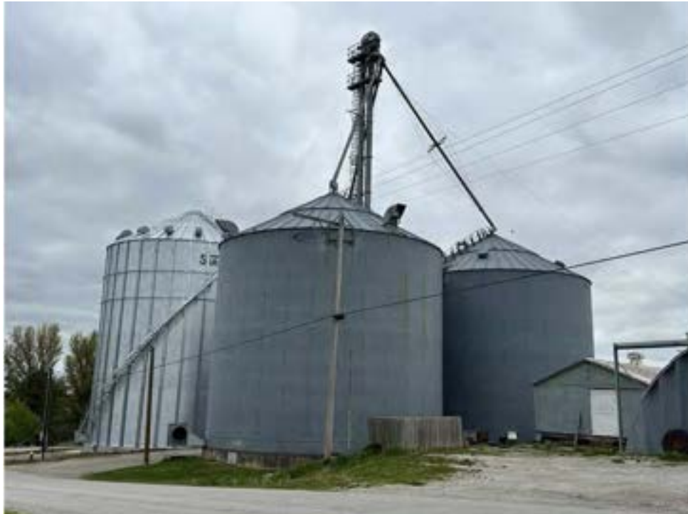
BELOW: Diagonal Grain Facility Sale Newer Sukup Bin constructed after the date of sale
