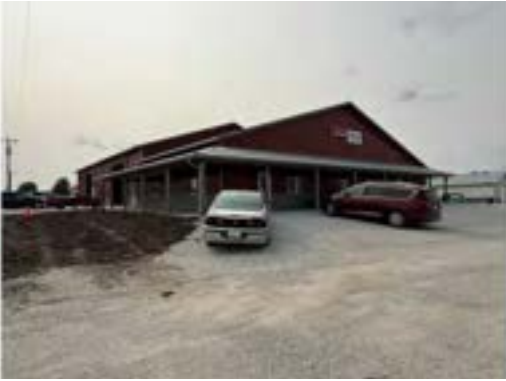
New Construction Building, Chariton Cost $64.86/sf Partial Commercial Quality Finish
