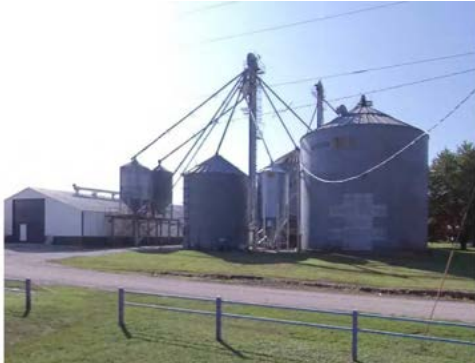
ABOVE: Seymour Grain Facility
