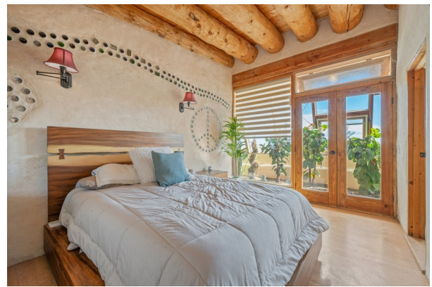
Bedroom: bottle-glass work & hand-troweled plaster
