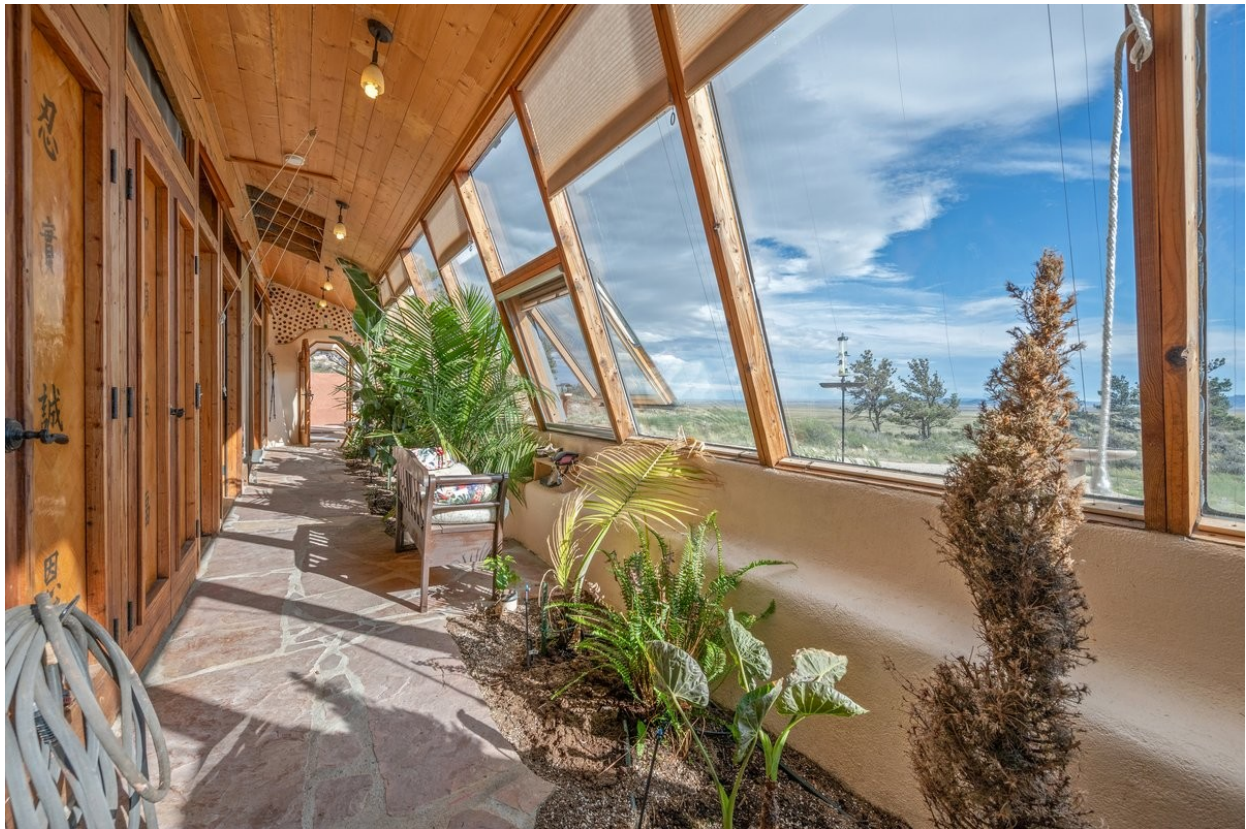
The greenhouse corridor: passive solar gain along the full south face
