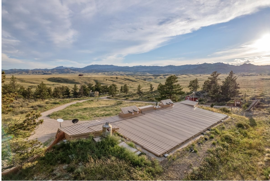
Generator shed, storage shed, and solar array from above
