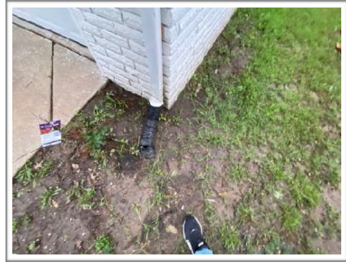
Existing gutter drain
