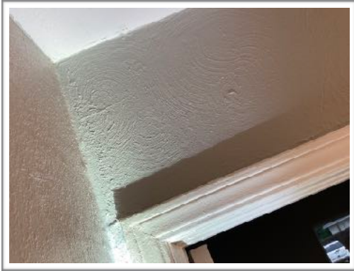
Repaired drywall crack
