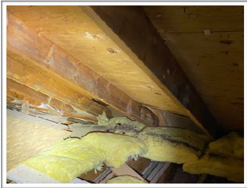
Attic, Roof framing
