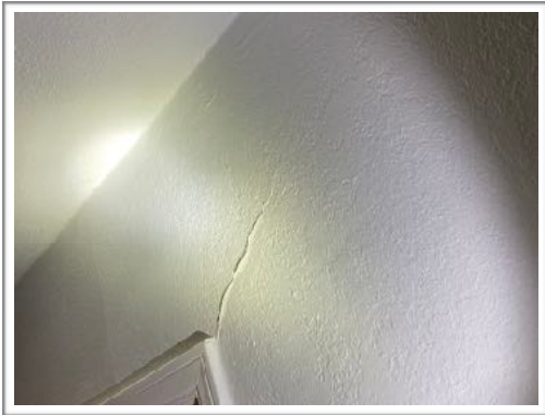
Repaired drywall crack
