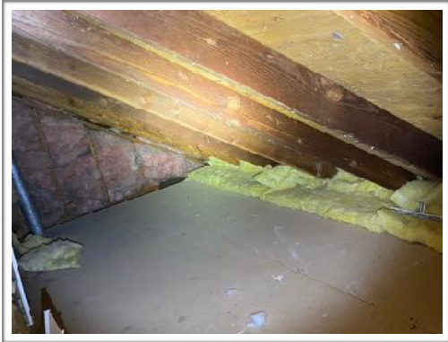
Attic, Roof framing
