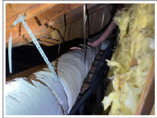
Attic, Roof framing
