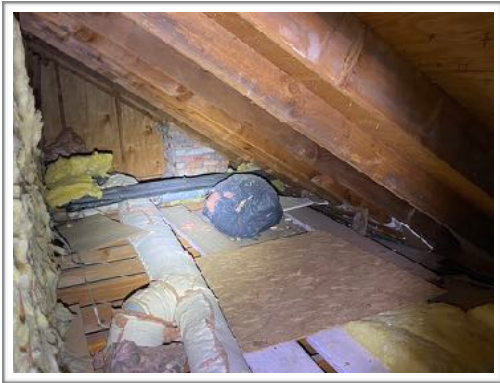
Attic, Roof framing
