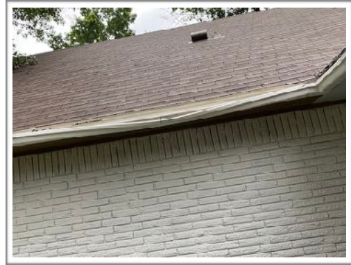
Damaged gutter
