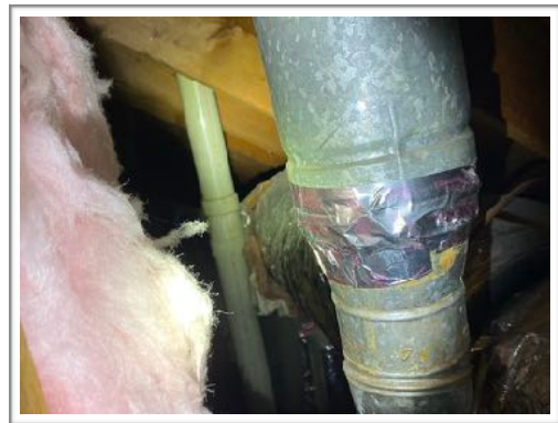
Attic, Roof framing
