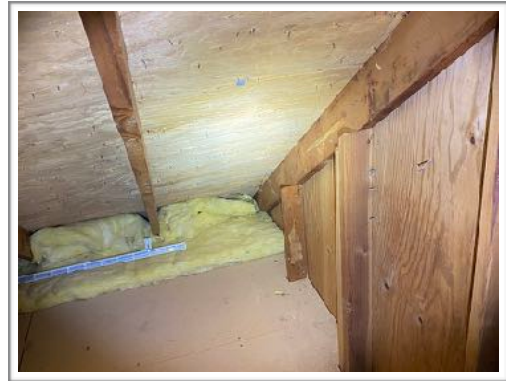
Attic, Roof framing
