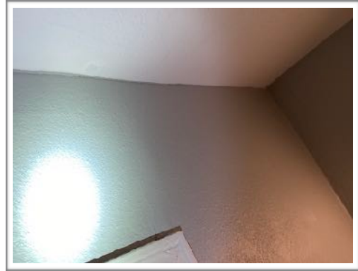
Repaired drywall crack
