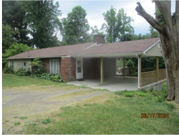
Main Structure Photo
